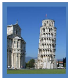
Leaning Tower of Pisa
